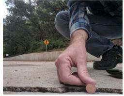
2) The roadbase near STA 18+00 (LT) is separating from the edge of pavement. This opening will allow runoff into the gap and eventually blow out the embankment.
