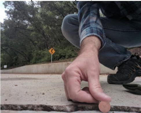
2) The roadbase near STA 18+00 (LT) is separating from the edge of pavement. This opening will allow runoff into the gap and eventually blow out the embankment.
